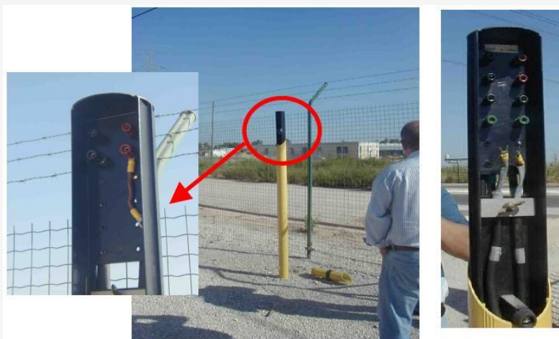
Figure 6.2 Cathodic Protection system
